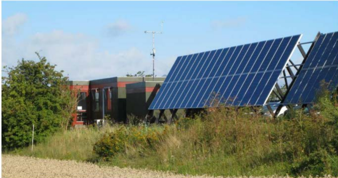
Figure 3: One PV plant located near building 715.
